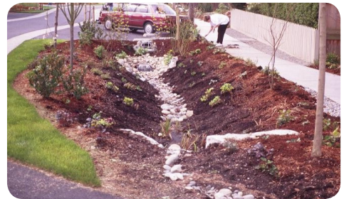
Bioretention Swales can include diverse plants, depending on site conditions.
